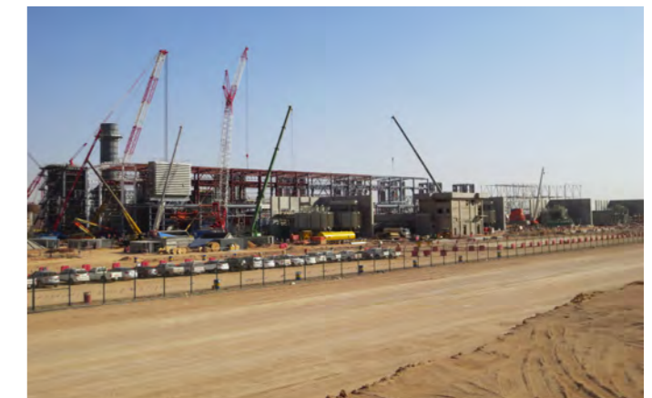
General View of Riyadh PP No. 12
