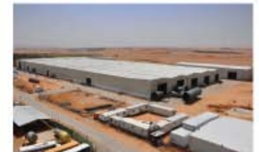
Steel Structure & Piping facility, Riyadh
