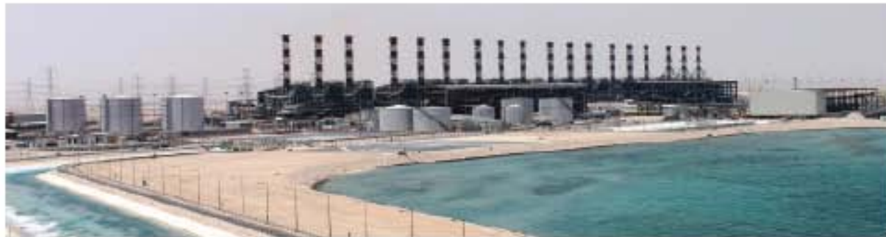
Overall look at Qurayyah Power Plant
